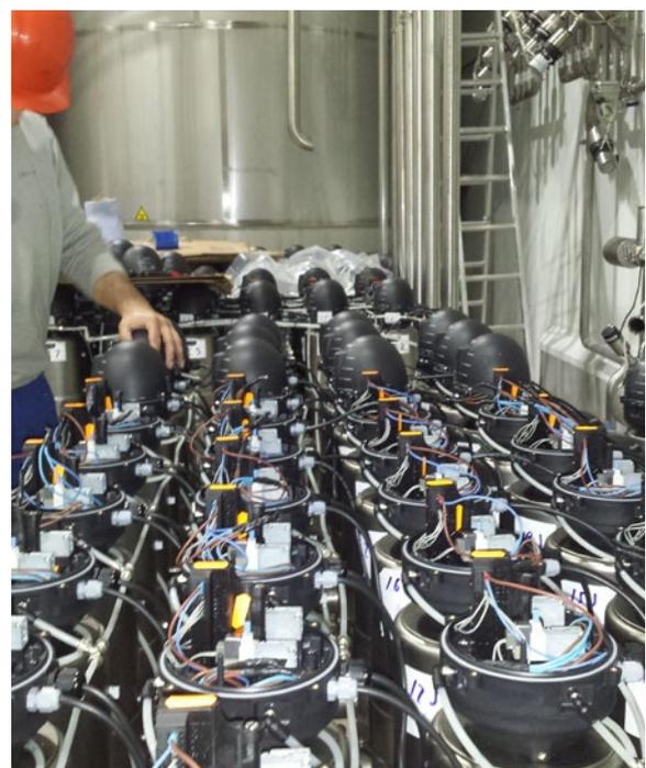
“ Automatic multiple system for the reception of raw material: Unloading of lorries by pump system, suction of liquid product in aseptic bag and pouring and grinding of frozen product”
