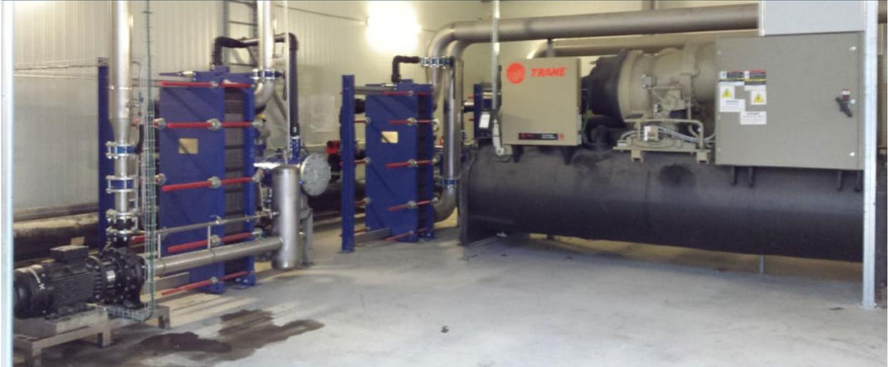
Exclusive system of refrigeration by sea water which was executed in the port and allowed to do without cooling towers and to reduce the energetic consumption of cooling equipments. A set of pumps installed in the seabed pump the water through a subterranean pipes system towards the services room where the water is returned to the seabed in a controlled temperature.
