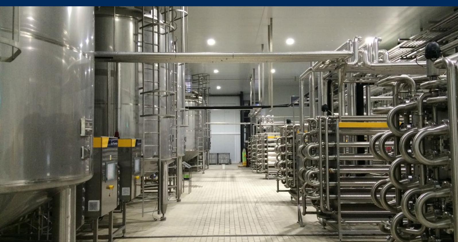
“ Six processing lines compounded by pasteurizer and aseptic tank. All the equipments are combined thanks to a completely automatic mixing room which has included recipes management and recipes control.
